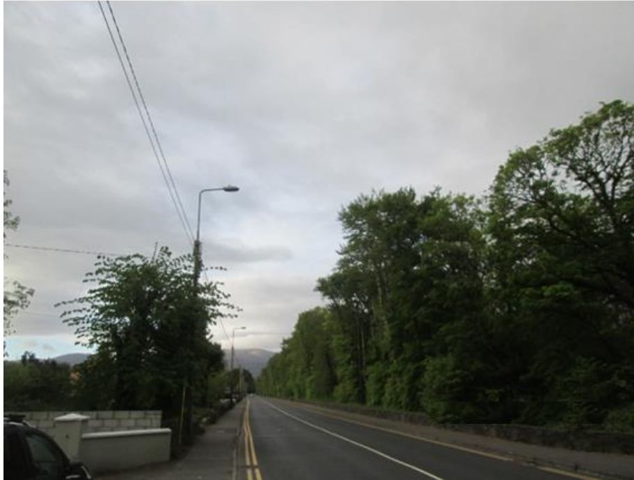
Photo 3: Existing Public Lighting on N71 (Port Road)
