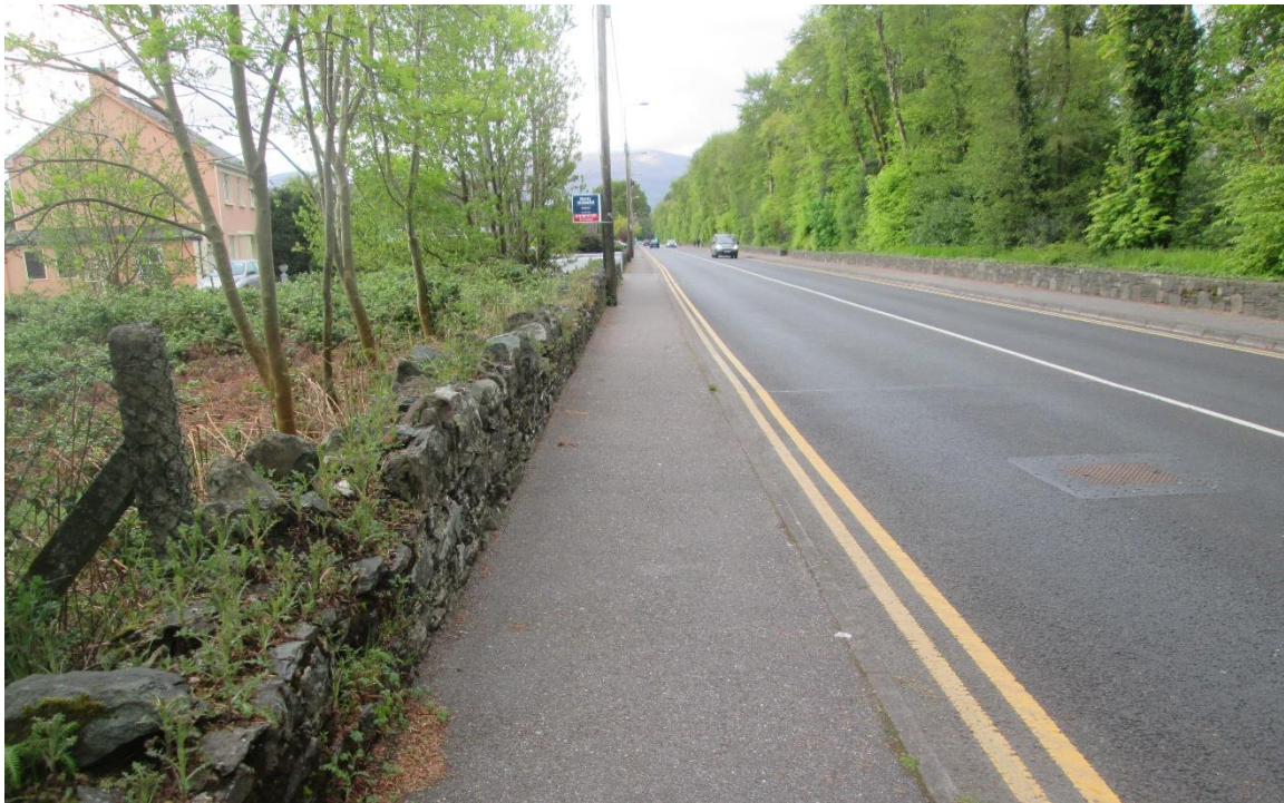
Photo 4: Existing Footpath along Eastern side on N71 (Port Road)
