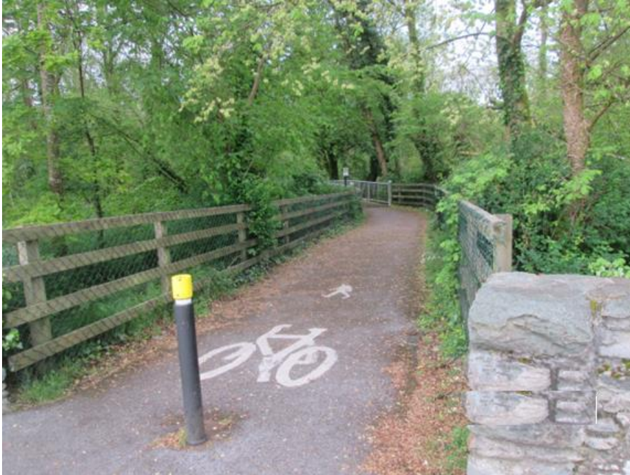
Photo 5: Existing Pedestrian/Cyclist Entrance into National Park
